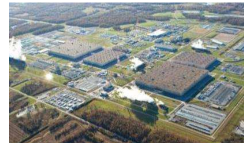
DOE assumed control of all facilities at PGDP to begin deactivation
